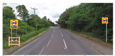
**Photo 11** – Relocation of terminal signs and Gateway panel incorporating village name.
