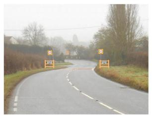
**Photo 10** – Possible gateway treatment at western entry to 30mph speed limit area
