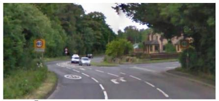
Photo 9 – Easternmost 40mph terminal signs under overhanging tree canopy.
